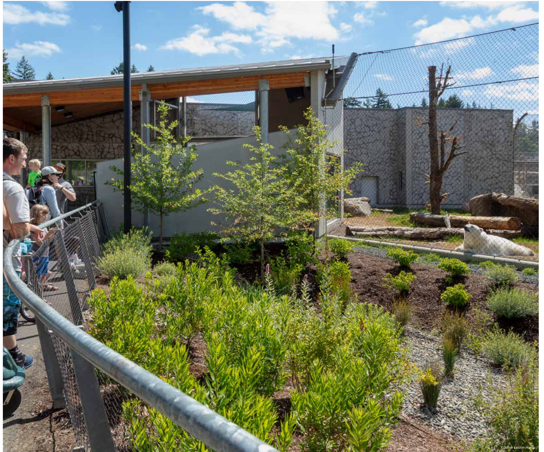
Green stormwater facility at Polar Passage
